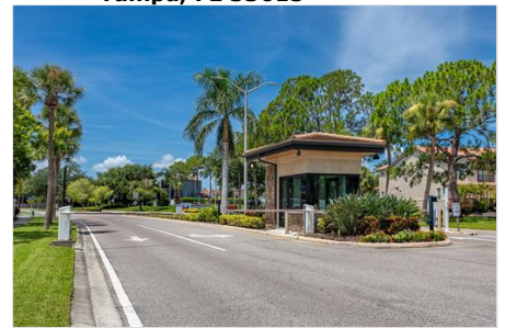
Front Gate-5936 Bayside Key Dr, Tampa, FL 33615
